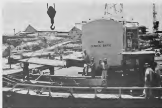
BY FITTING this steel plate over the engine compartment, the fire boat can be quickly converted into a work boat when needed. The boat resulted from tremendous co- operation among Marine, TSD and Mechanical personnel. DOOR DI instala e planchi di stal aki ariba e compartimento di motor, e boto di can- dela por worde rapidamente converti pa un boto di trabao ora ta necesario. E boto ta resultado di un tremendo cooperacion entre personal di Marina, TSD y Mechanical Dept.
